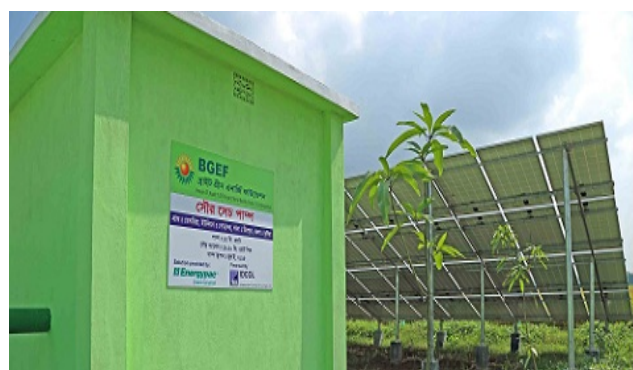
Solar Irrigation Pump Installation in a Bangladeshi off grid area
